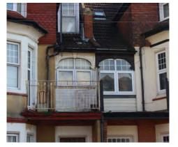
An example of poorly maintained balconies, the one on the right has been lost entirely
